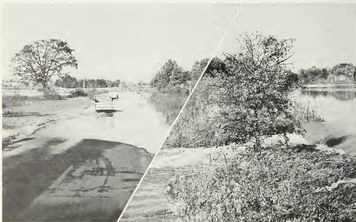
Levee failure and inundation of roads frequently cause losses along Big Creek.
